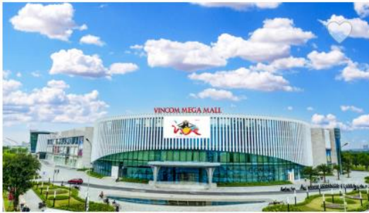
VINCOM MEGA MALL SMART CITY
