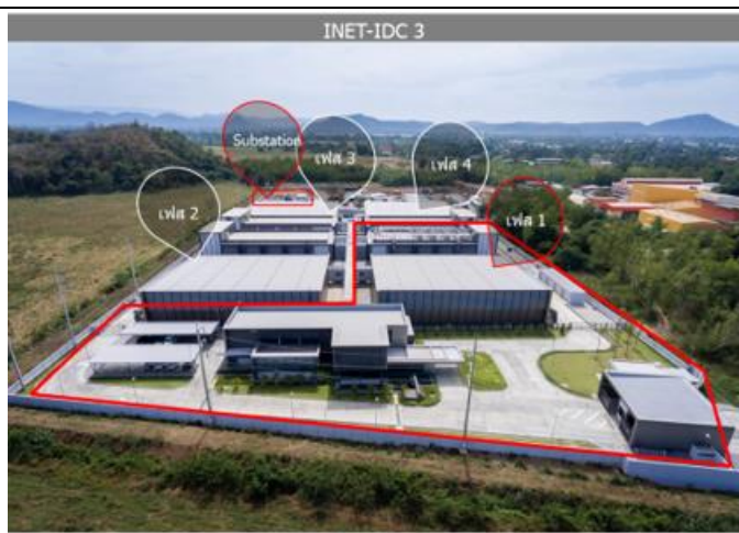
Figure 1: Invested assets - INET-IDC3 Phase 1 and substation
